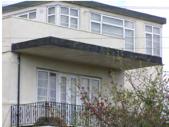
Picture 4.48 First floor balcony to number 8 Valencia Road
