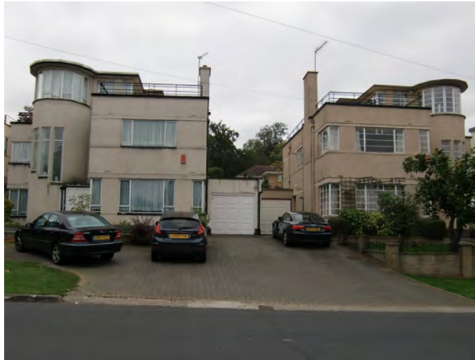
Picture 4.44 Number 4 (right) remains closer to the original Modernist design than number 6 due to the retention of original Crittall windows
