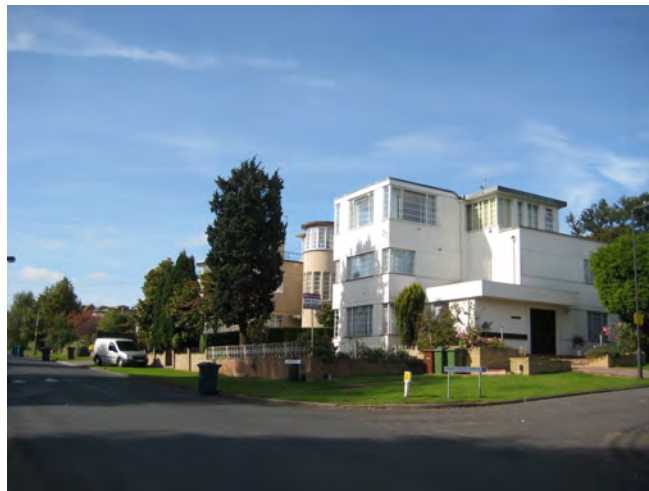
Picture 4.1 View towards Number 2 Valencia Road demonstrating the Modernist Style set off by plentiful greenery that characterises the Conservation Area
