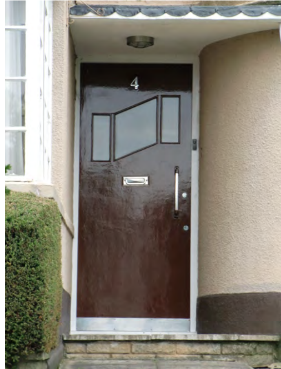
Picture 4.90 Strong geometrical shapes to the door of number 4 Valencia Road complements the Modernist style
