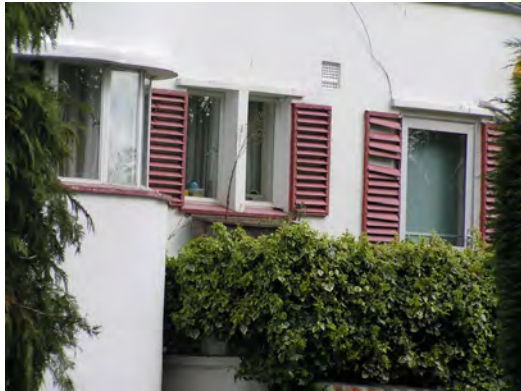
Picture 4.85 Original shutters on number 4 Kerry Avenue
