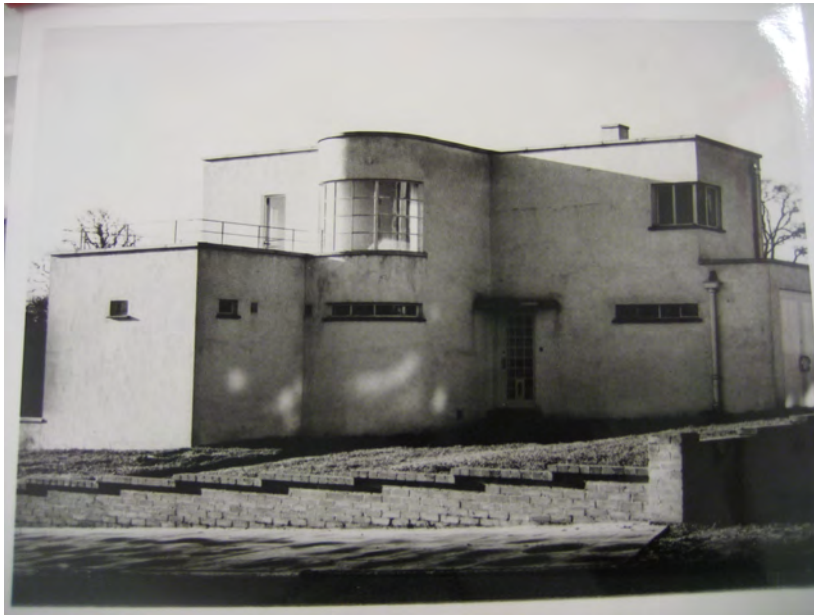
Picture 4.11 Number 5 Kerry Avenue As Built, Pictured 1937 (View from the West)
