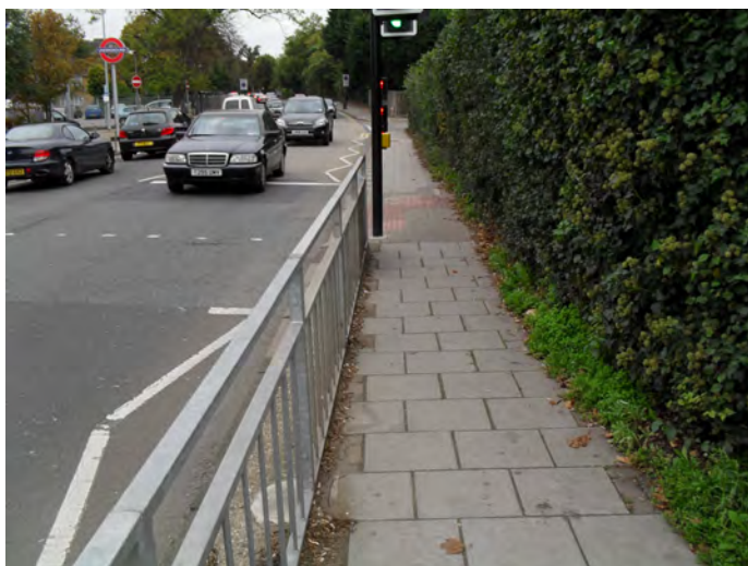
Picture 4.19 The high hedge between London Road and Kerry Court does much to shield the
