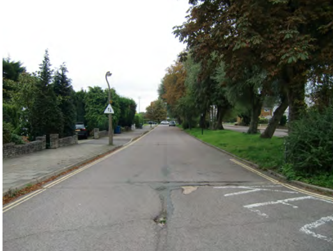
Picture 4.93 Low boundary walls do help to unify the lower east side of Kerry Avenue
