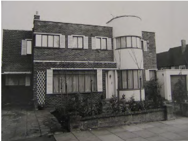
Picture 4.57 Number 2 Kerry Avenue before some of the modern alterations to the building (date of photo unknown)
