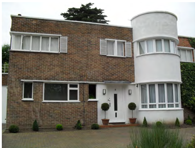
Picture 4.5 Number 3 Kerry Avenue, like other buildings in the Conservation Area, is one of the earliest domestic group in west London to adopt the principles of the Modern Movement
