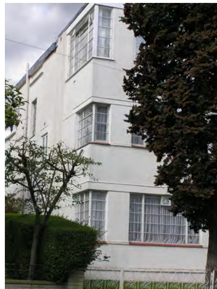
Picture 4.79 Original Crittall windows on number 2 Valencia Road
