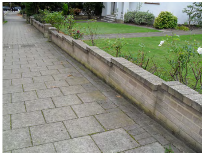
Picture 4.97 Original low boundary treatment to number 5 Kerry Avenue looking southwards
