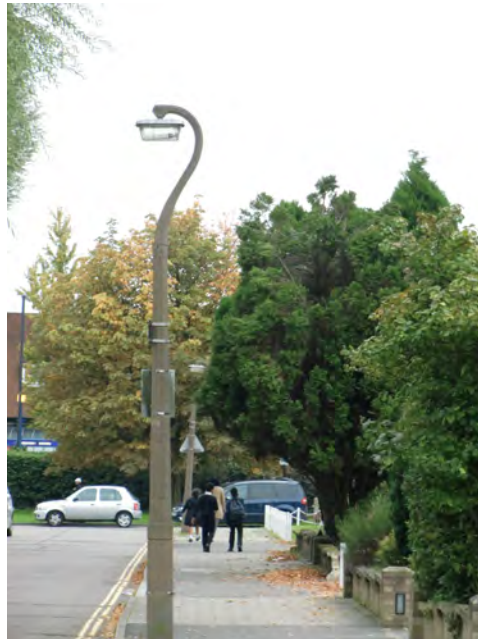
Picture 4.110 Original concrete street lamp on lower Kerry Avenue complements the Modernist designs of the area
