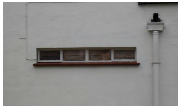
Picture 4.83 Flat window on number 5 Kerry Avenue
